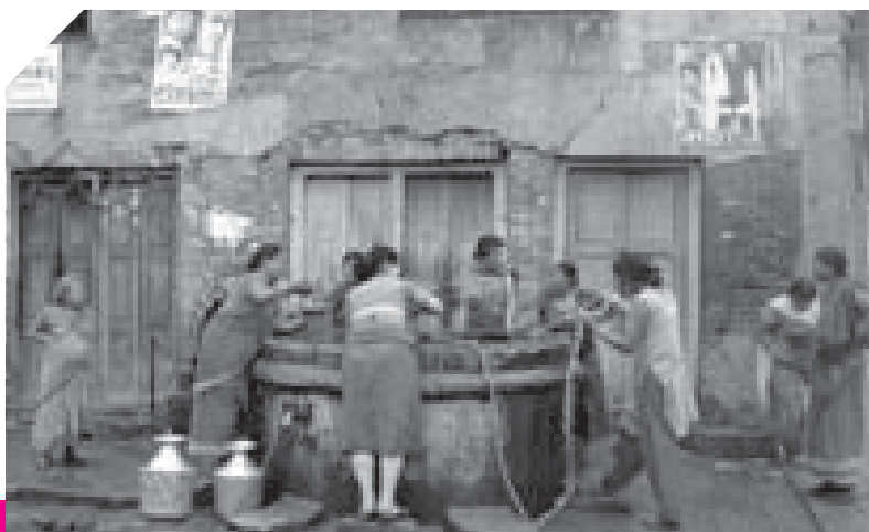
Tun , the typical traditional public dug well
