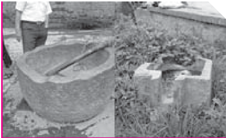
The stone flow distributors at Mangā Hiti and Sincha Hiti, left unattended after its replacements in recent time
